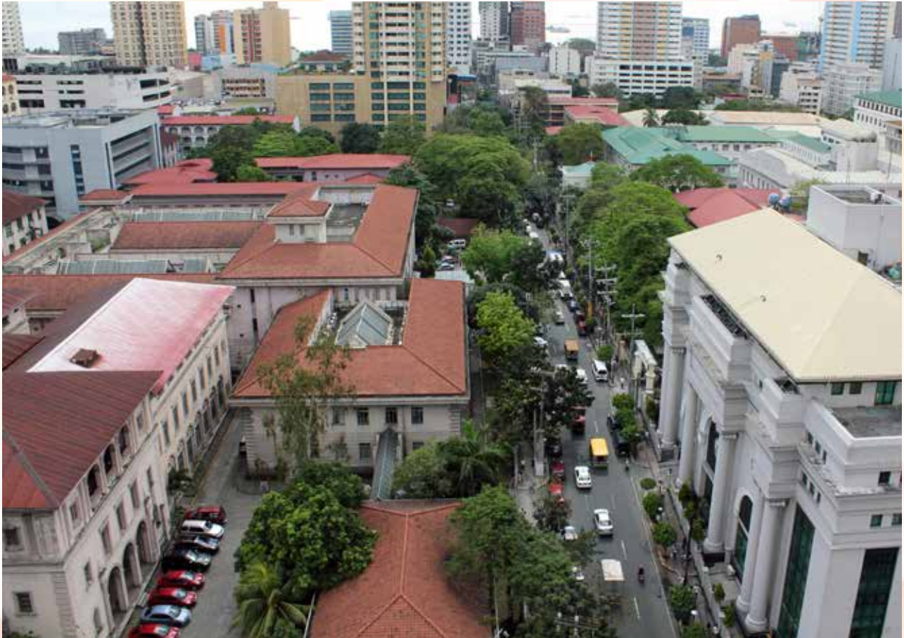
Aerial view of UPM-PGH showing entry points along Padre Faura street
