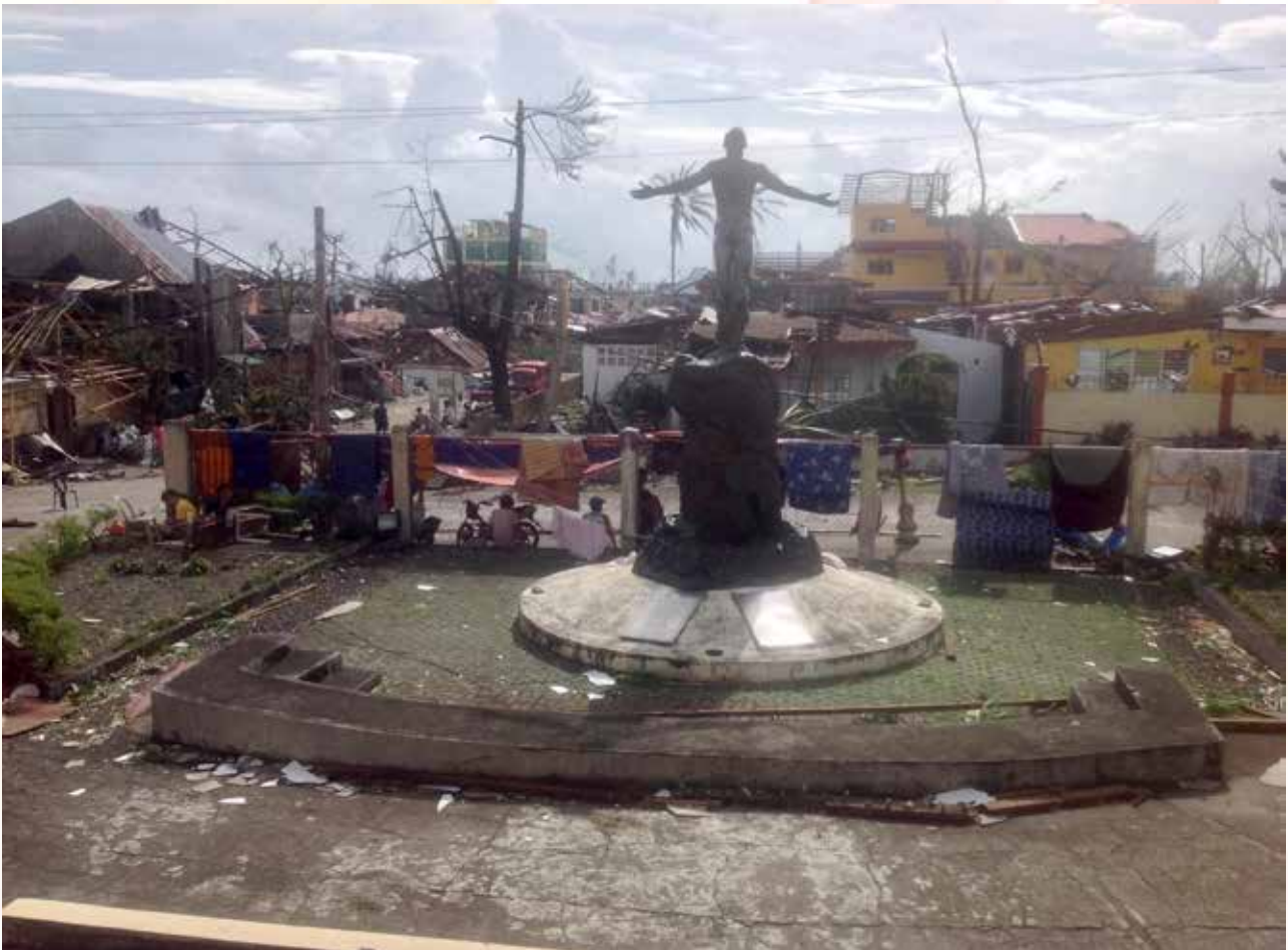
Part of the damaged campus of SHS Palo, Leyte
